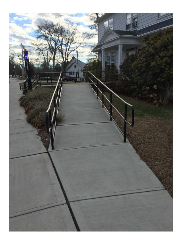
This feature contains Concrete Ramp. There are Ramps/Walkways 5 feet wide and approximately 30 | Total Area: 150 square feet. feet total length.
