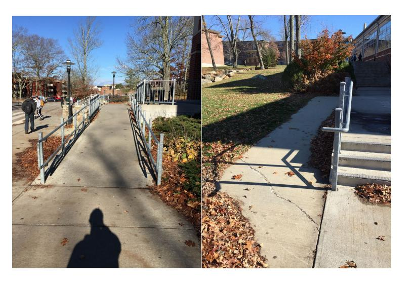
This feature contains a Concrete Ramp. There are Ramps/Walkways 5 feet wide and approximately | Total Area: 165 square feet. 33 feet total length.
