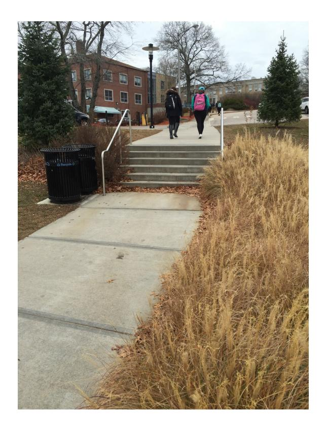
This feature contains 2 sets of concrete stairs with a large plaza in between, and a landing area at the doorway entrance. The upper stairway has 6 stairs @ 28 ft wide. The lower stairway has 5 stairs @ 25 ft wide.
