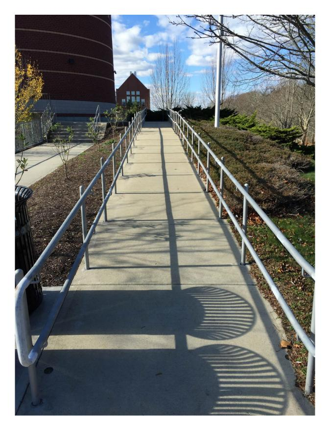
This feature contains a Concrete Ramp. There are Ramps/Walkways 5 feet wide and approximately | Total Area: 150 square feet. 30 feet total length.
